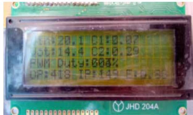
LCD readings during on load operation
